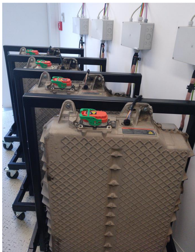
Figure 2: ELSA second-life lithium ion battery packs installed at the RWTH Aachen pilot
