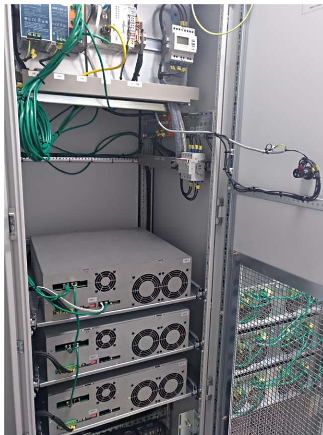
Figure 1: ELSA DT5 system power electronics and controllers installed at the RWTH Aachen pilot
